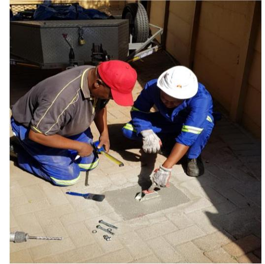
Fit the two anchor bolts through the Anchor Point product and fit the washers and the two nuts. Tap it into the drilled holes and push the Anchor Point into its position. Using the hammer, tap the bolts down until it becomes flush with the product. Tighten the nuts with 19mm socket until tight. Remove the nuts and fit the shear bolts and tighten until the top section of the nuts break off.
